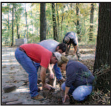
Marcus Orf, Lane Lenderman and Eddie Hendrix placing blocks along the walkway.
