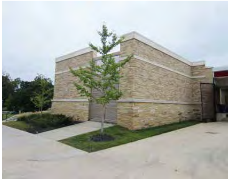
Appropriate Screening for Utilities
