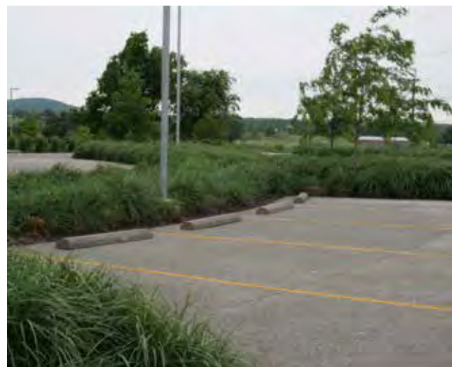
Pervious Concrete Paving
