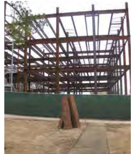
Existing Building Under Construction
