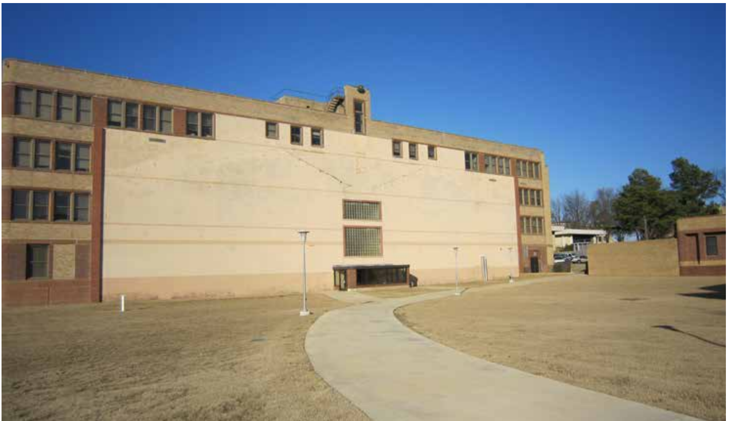
South facade of Business Building
