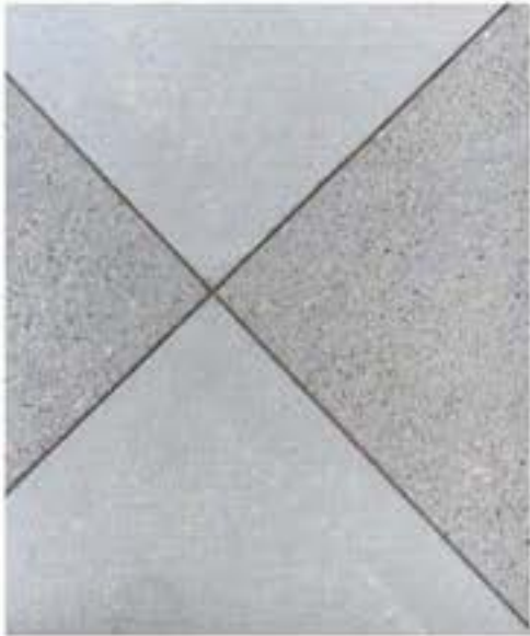
scored and lightly sandblasted concrete
