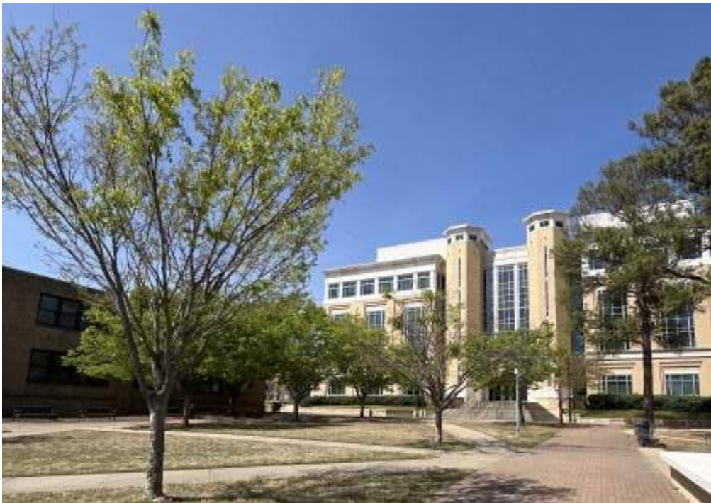
6. WIDESPREAD DISEASE AND MAINTENANCE ISSUES
