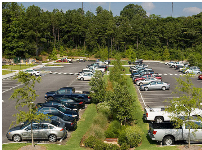
A bioretention area is located in the center of the parking lot to capture stormwater.
