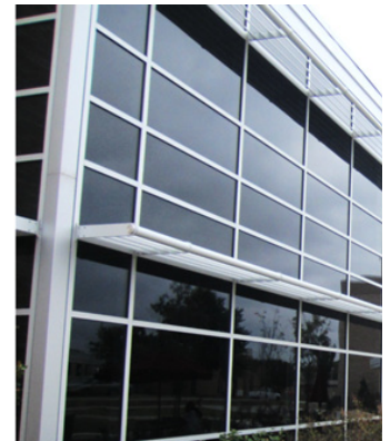
Curtain Wall Windows
