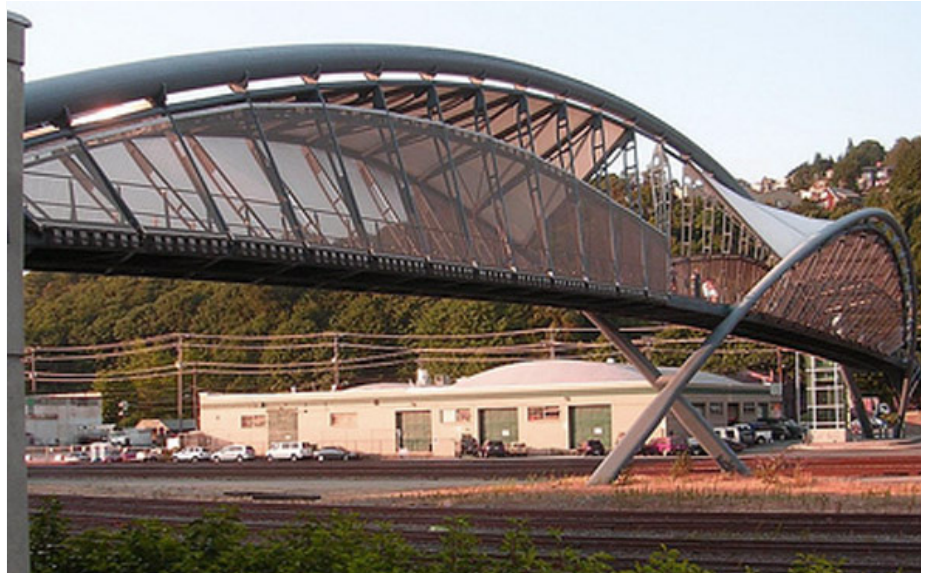
Pedestrian crossing over railroad tracks Elliot Avenue Helix Bridge, Seattle, WA
