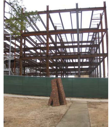
Existing Building Under Construction
