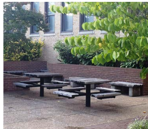
Existing non-conforming wood and metal picnic tables in deteriorating condition.
