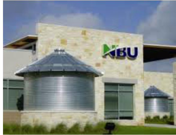
Above ground cisterns can be visually appealing and used as educational tools
