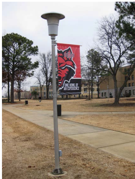
Non-conforming fixture with banner mount attached.
