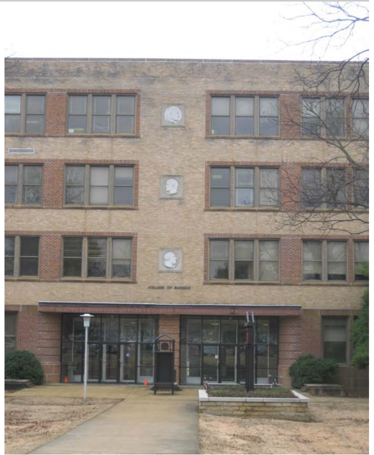
North facade of Business Building
