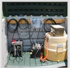
Edge-of-field monitoring utilizes high-tech sensors to assist producers in water conservation by providing practical tools such as remote pump management.
